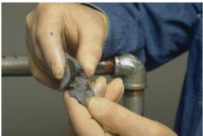
Knead together the inner and outer core of FIX STIX™. If mixing is difficult, warm to
