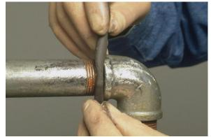
4. Apply FIX STIX<sup>™</sup> to damaged area. Fill in holes, cracks or offsets.
