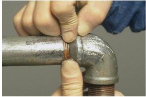
5. Press FIX STIX<sup>™</sup> firmly into the damaged area to ensure a solid fill.
