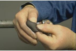
3. Ensure FIX STIX<sup>™</sup> is completely mixed and the color is a uniform dark gray.
